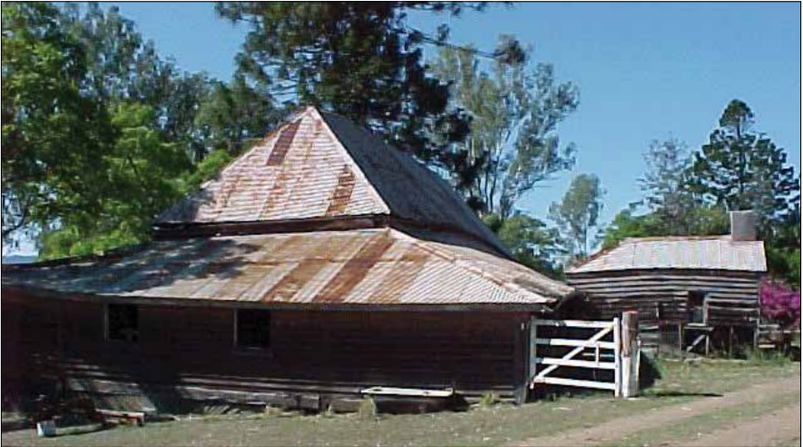
The woolshed prior to the demolition of the old kitchen. Image courtesy Margaret Hockey and Nathanael McGhee.
